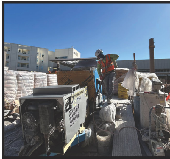
Journeyman, Johnathon Houser working at Hoag Hospital
